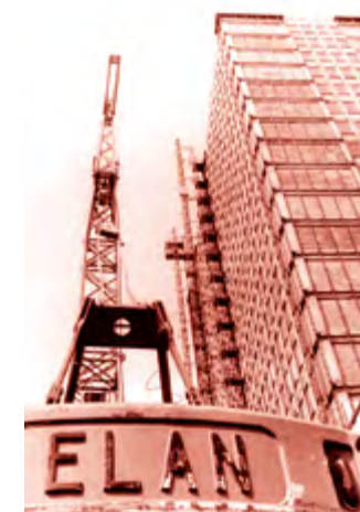
Stavba budovy A1 Construction of the building A1
